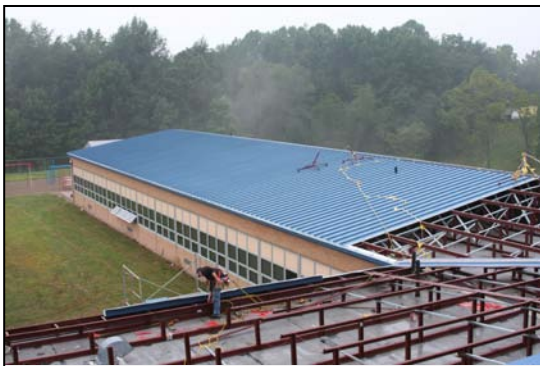
New Sloped Metal Roof over Existing Flat Roof
