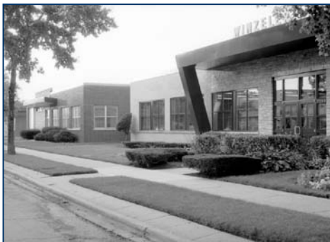
Wall Retrofit - Before
