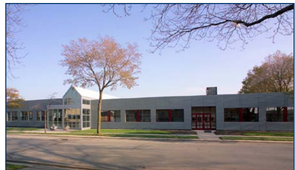
Wall Retrofit - After
