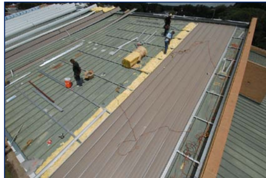
New Metal Roof over Existing Sloped Metal Roof
